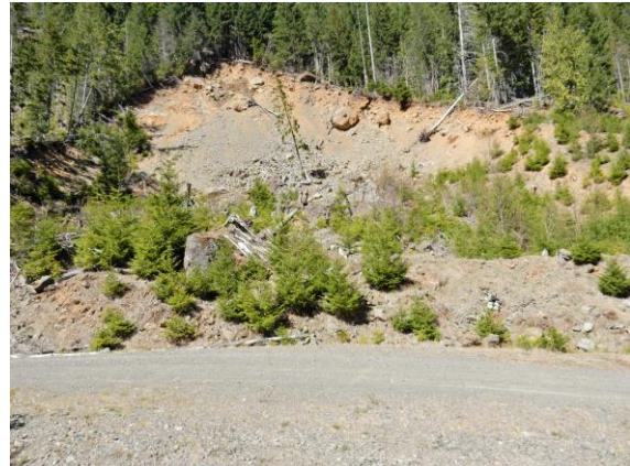
Photo 4: Newer slide 3 (circa 2017) which has its headwall above the road, and the slide was observed to have crossed Wilfred Creek during the failure event.
