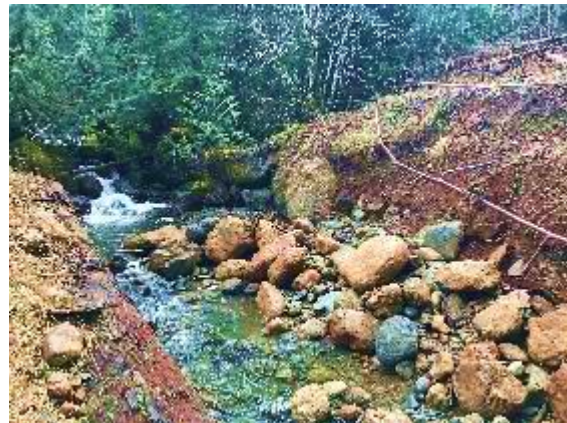
Photo 8: Cowie Creek deactivated bridge site with exposed side banks.
