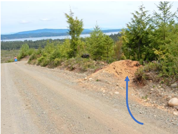
Photo 7: Example of good road maintenance practice in making diversions drains graded into the side cast, on private roads – Hastings Main.
